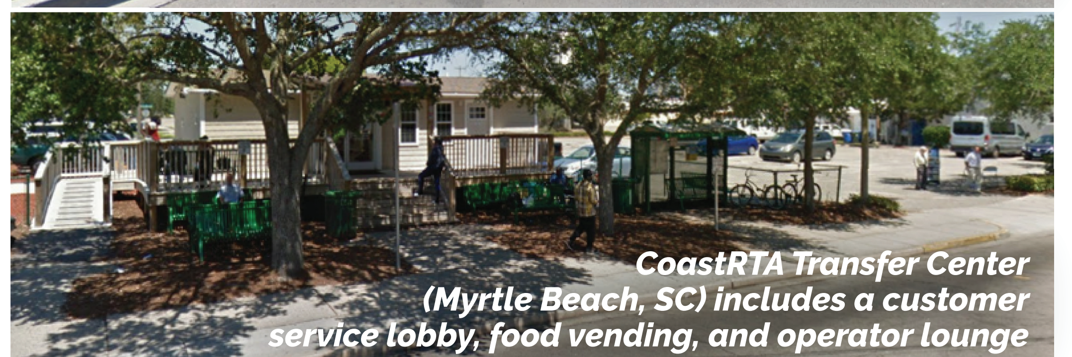
Roam Transit Hub (Banff, Alberta) includes seating and shelter that features local architecture, wayfinding, real-time arrival information, and an in-lane stop for buses
